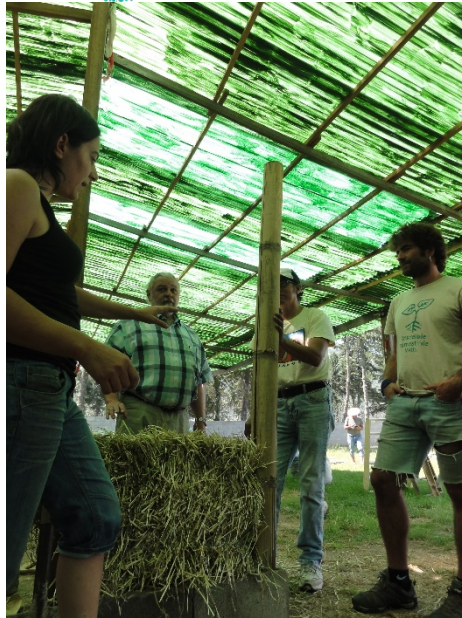
Showing the technique used in the house construction
