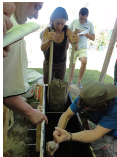
ramming the prepared earth
