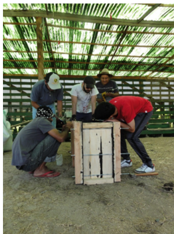
Preparing the mold for the rammed earth
