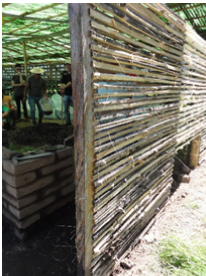
Structure ready to receive the mixture
