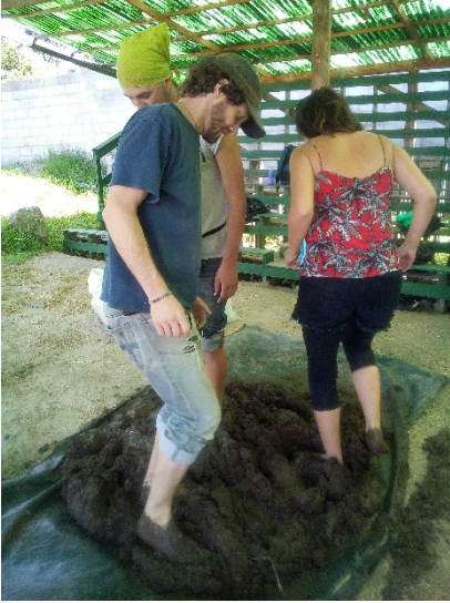
Preparing the mixture for the plastering
